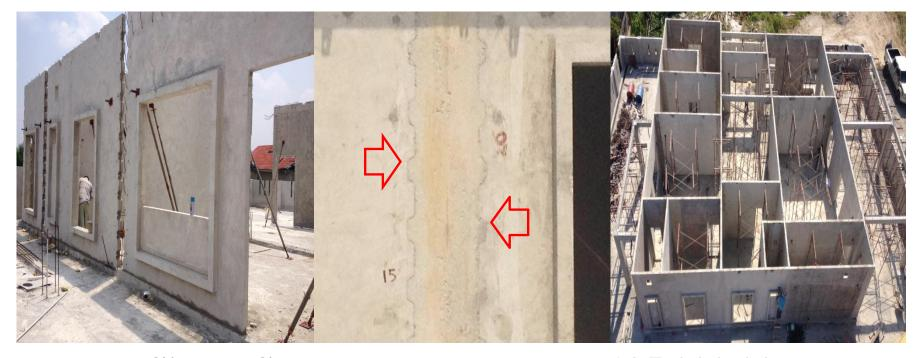
Single Storey Bungalow RM 125,000.00 3,891.31 ft2 / Wall High 4.0m / R.C Flat Roof Completed In 10 Days With 6 Workers Precast Element 86 %, Wet Work 14 %
